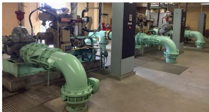
Fowle pump station pumps 1.5 million gallons of water per day from Freedom reservoir and sends it through our pipes for distribution. It is 50 years old and will need to be replaced in the next 5-10 years.
